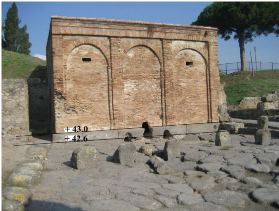
Figure 2.2. South façade of Castellum Aquae with indications of levels for the three openings. The middle one slightly above and the left and right ones are on the same level. Photo and indication of levels by author.
