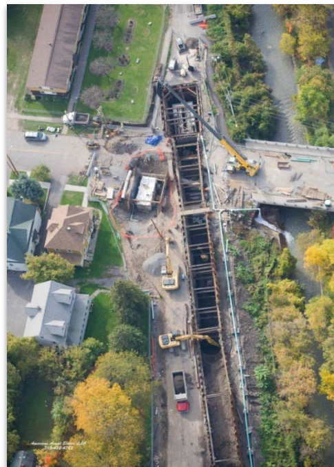
Figure 3-3: Construction at South Avenue & West Castle Street Intersection
