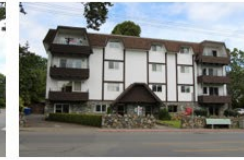
ADJACENT EAST PROPERTY FROM OAK BAY AVENUE
