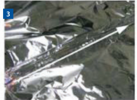
3 Lift the overlap, crease and fold flat for the length of the seam (26").
